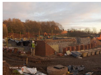
The start of Brickwork to the building
